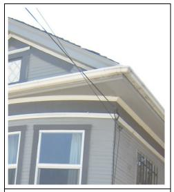
Figure 6 Level soffit at ceiling height. Note wide band between soffit and tops of windows. Photo: John Fryer, GGASHI
