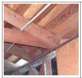
Figure 1 GOOD: Typical roof rafter connection to wall and ceiling joist used in contemporary construction. The ceiling joist ties rafters on opposite sides of the house together so the walls do not spread apart. The "face-nailed" connection from the joist to the rafter is the most secure type of nailed connection.
