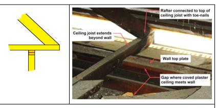
Figure 3 **BAD:** Archaic roof connection using extended ceiling joists to create soffit at eaves. The rafter connection to ceiling joist is marginal. Photo: Max Curtis, GGASHI
